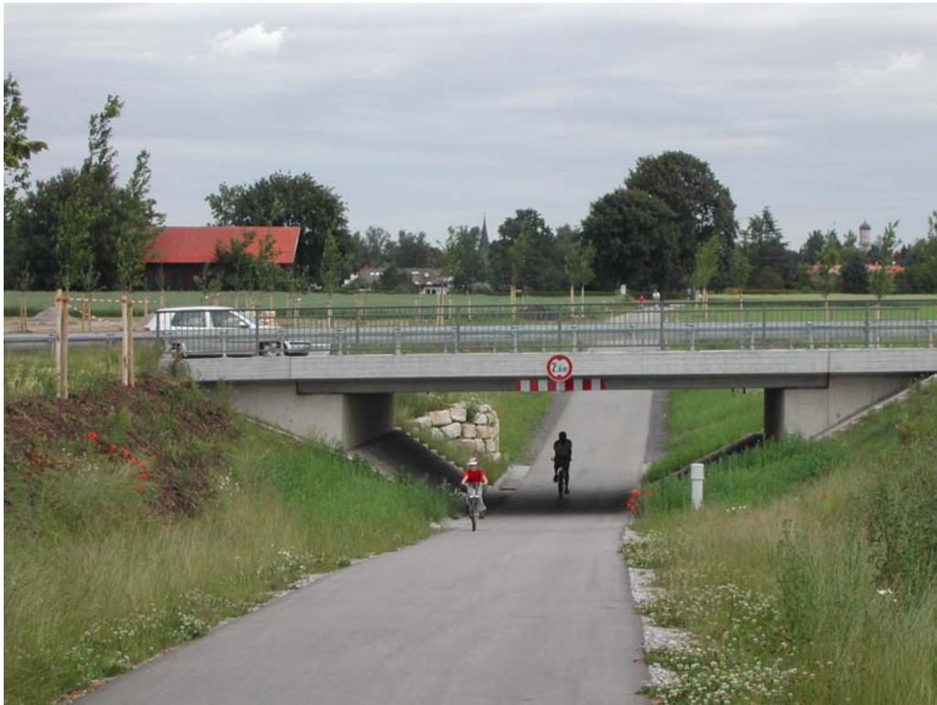
Figure 6: Roadside Trail Underpass, with Steps to Road on all Four Sides
